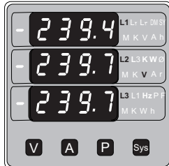
Screen : 1 Voltage Line to Neutral (For Ph r Wire only)
