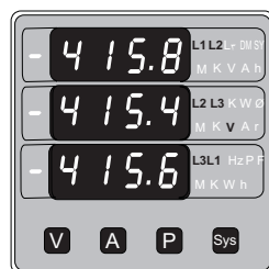
Screen : 2 Voltage Line to Line (For Ph r Wire r & Wire)
