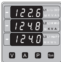
Screen : 5 Phase Apparent power (For Ph r wire only)
