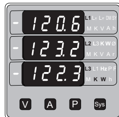
Screen : 4 Phase Active power
